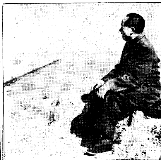
Inspecting construction on Yellow River in 1952
