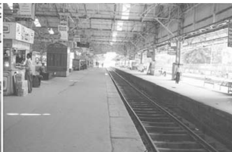
Sealdah Station, Calcutta at 9-45 a.m.
